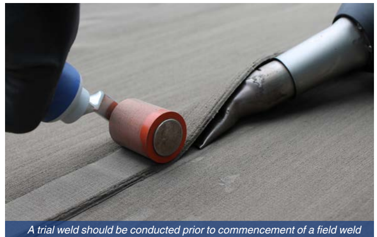
A trial weld should be conducted prior to commencement of a field weld
