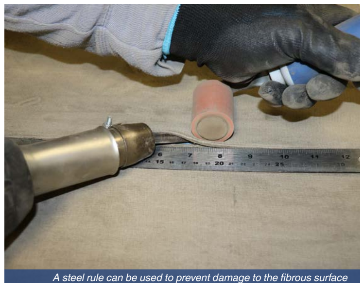
Weld Track C would need to be opened carefully to access Weld Track B
